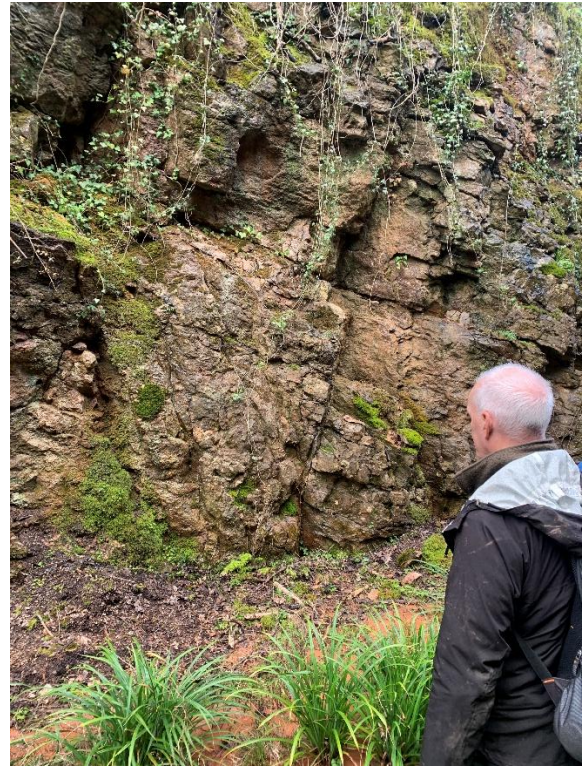
Conjugate fault in cutting wall
